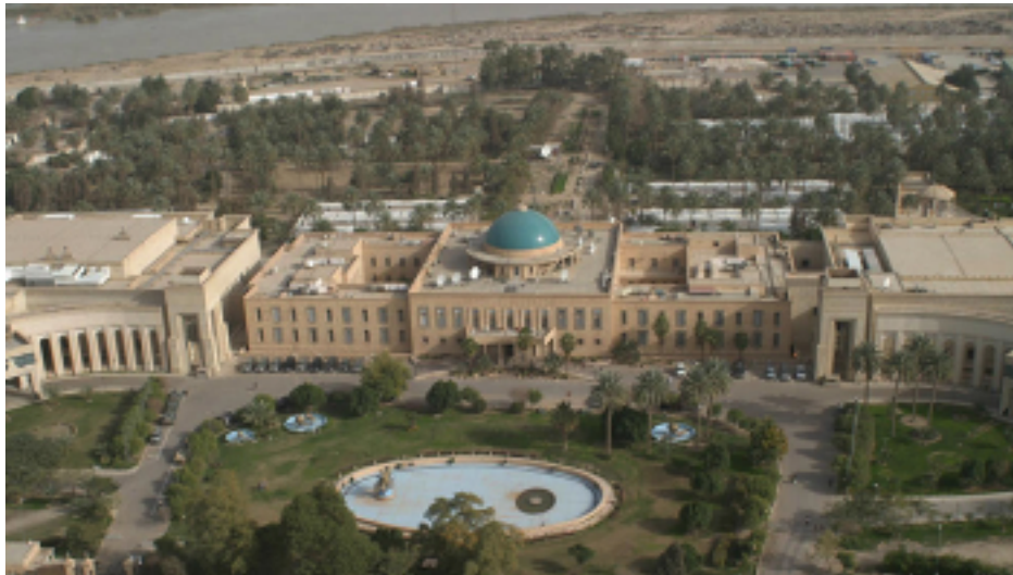
U.S. Embassy compound in Baghdad's Green Zone
